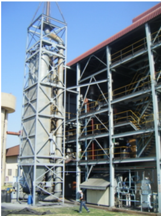
Figure 3b: Combustion test facility building
